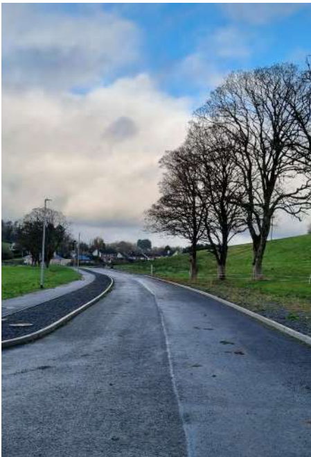
4. Existing site access under construction
