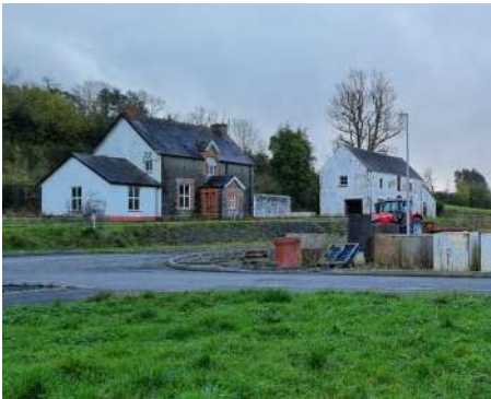
5. Existing derelict buildings along access road
