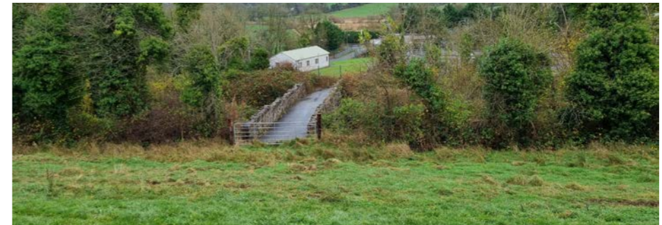
10. Existing footbridge to Railway Walk
