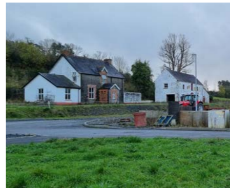
5. Existing derelict buildings along access road
