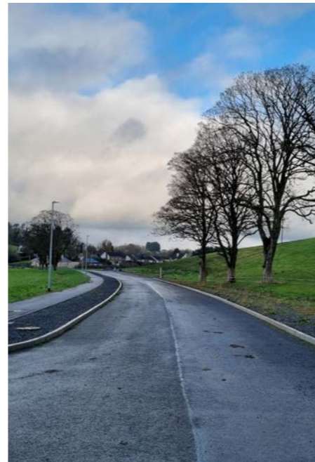
4. Existing site access under construction
