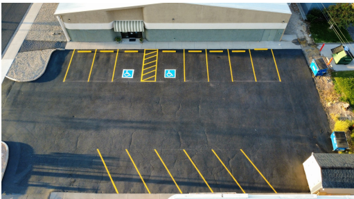
Small commercial lot. Fresh seal coat, bright yellow striping, two ADA spaces marked to code.
