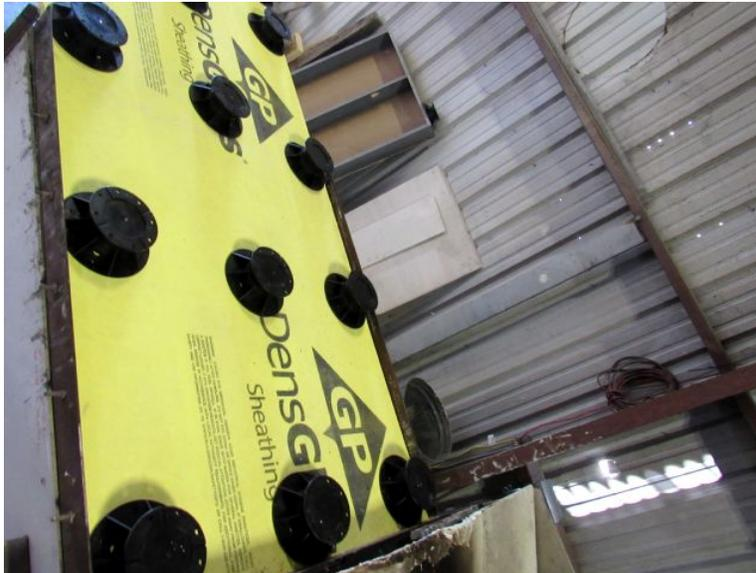
**Top View: Adjustable plastic leveling pedestals resting on GP DensGlass® Sheathing**
