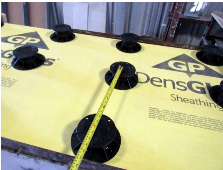
**Adjustable plastic leveling pedestals spaced 16 inches apart in the width direction and 24 inches apart in the longitudinal direction.**
