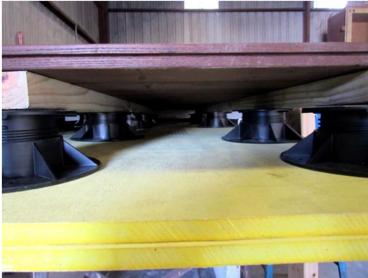
From bottom up: Two layers GP DensGlass® Sheathing, adjustable plastic leveling pedestals, 2 x 4 board runners and the Thermally Modified Ash Decking Panels
