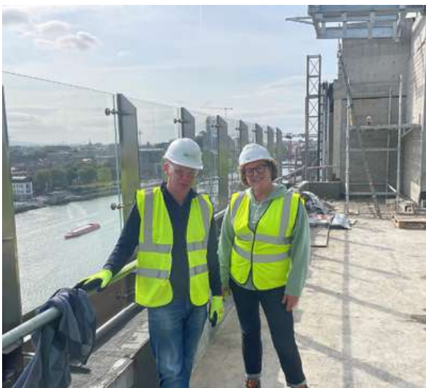
IGBC 25 North Quay Wall Site Visit
