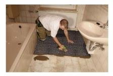
6. Put in **DAMTEC® multi** without fold and rub and press carefully. For the second half work in same way.
