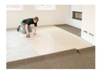
**4.** Fold back **DAMTEC® multi** to the middle of the room and glue the underlay to the substrate, observing the instructions of the adhesive and floor finish manufacturers.
