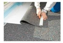
**3.** Use a regular carpet knife in conjunction with a steel straightedge for cutting to size.
