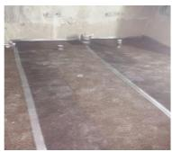
Also possible but not recommended using the mat as the peripheral insulation strip. This is under responsibility of the installer and it has to be ensured that the minimum thickness, especially at the edge, is not less than necessary. This is only possible for mats less than 8mm. To have a rectangular angle in the corner of the edges, it is useful to cut the mat.
