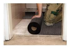
3. Place **DAMTEC®** multi over the entire surface to be covered. Trim to size slightly larger than the surface covered. Leave the underlay in place for one day to allow dimensional relaxation and temperature equilibration.
