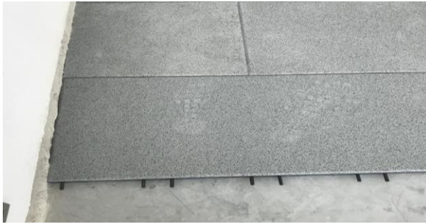
Each row should be offset by a half tile;
