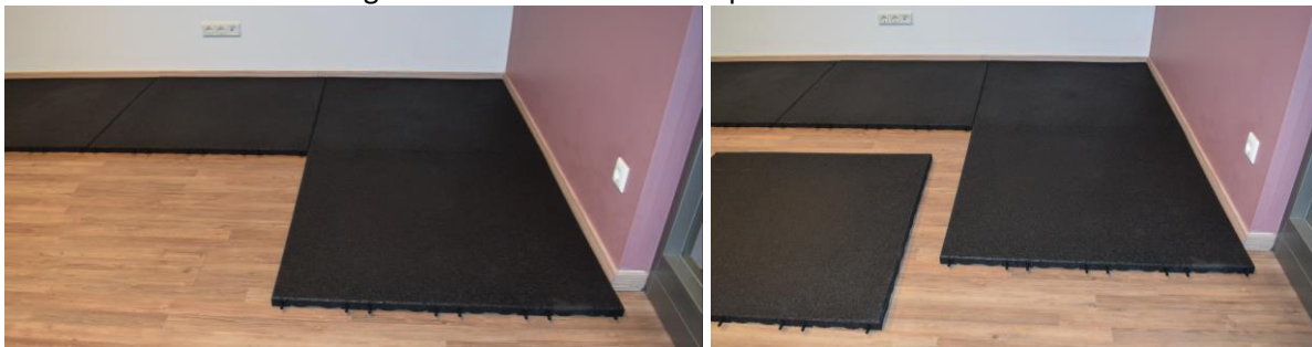
Start the second row of the tiles in the same way and continue; place the tiles next to each other
