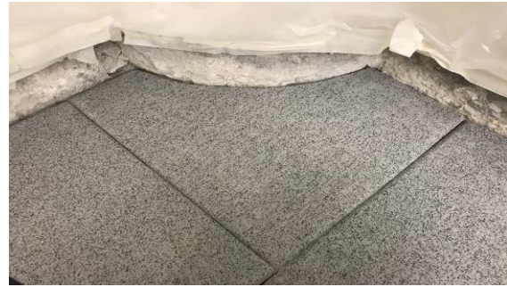
tiles can also be cut around curves
