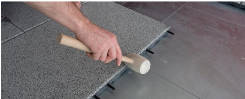
Closing the gaps with a hammer
