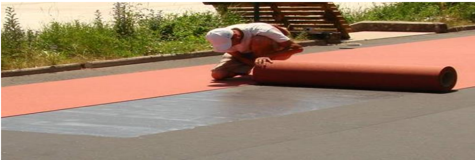
Rolling out the top layer over the elastic layer
