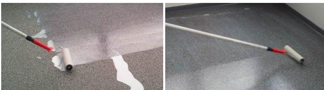
Applying of the coating
