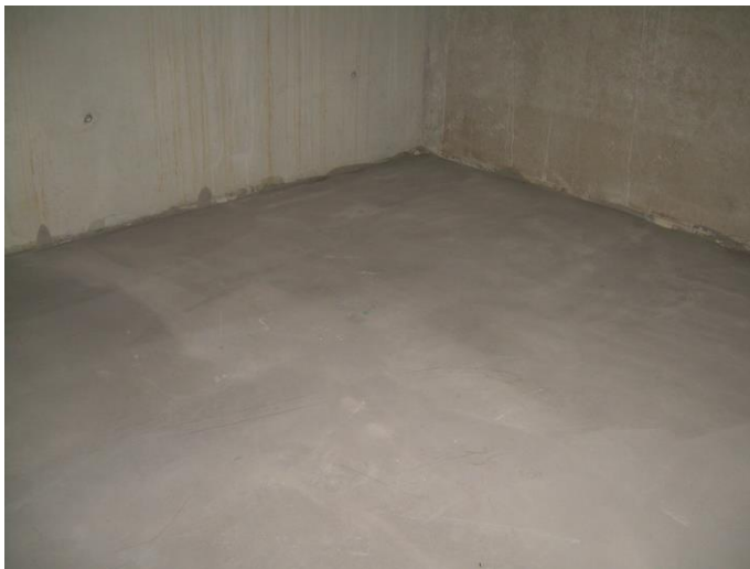
Even, suitable substrate made of poured screed
