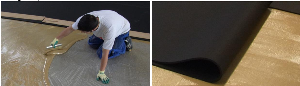
Adhesive application to clean substrate; roll out into the adhesive bed
