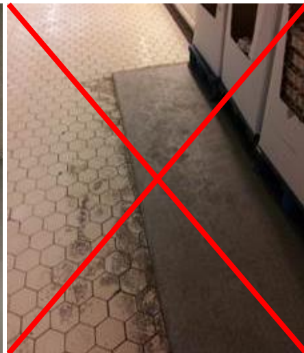
not suitable substrate
