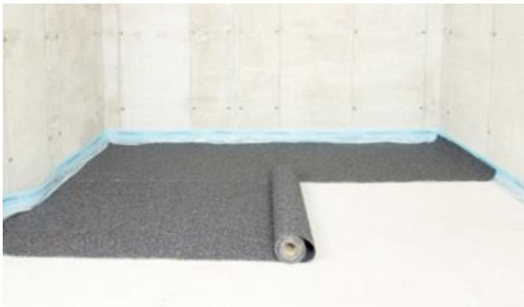
Installation of the individual rolls joint to joint
