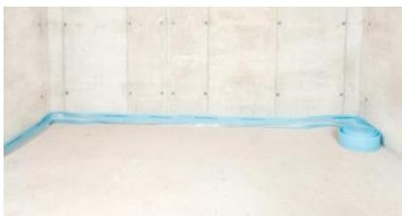
Installation of an edge insulation strip
