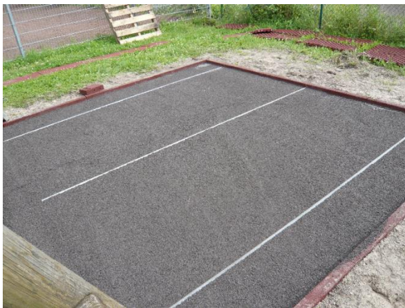
Levelling crushed sand/stone chippings
