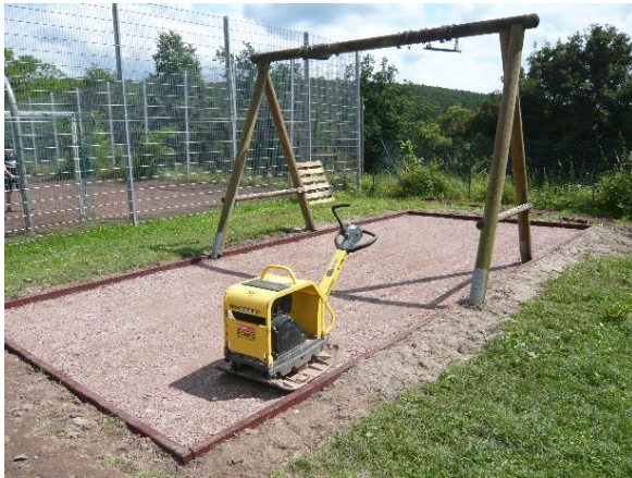
Crushed stones bed stable compacted
