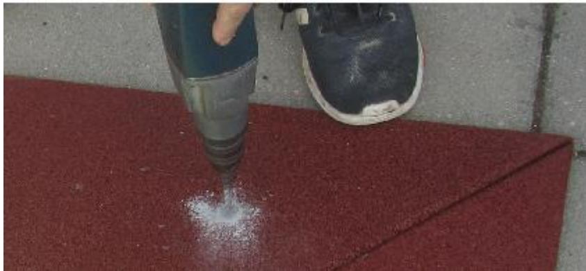
The screw head should be countersunk as deeply as possible within the profile.
