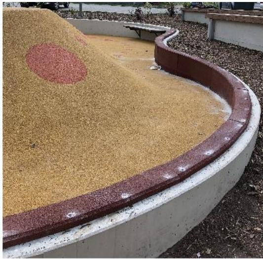
For this purpose, the angle elements are glued across the entire surface and additionally secured in a force-locking manner using countersunk concrete screws. The surfaces of the countersunk heads may also be sealed with polyurethane adhesive.
