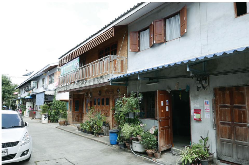
Photo 3: Housing improvements based on communities' input
