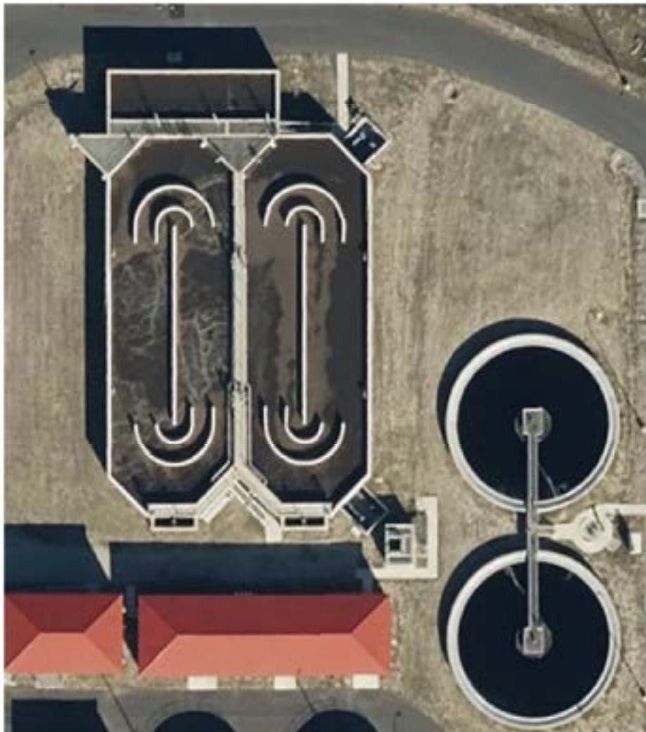
Dual Continuous Loop Reactors with Clarifiers
