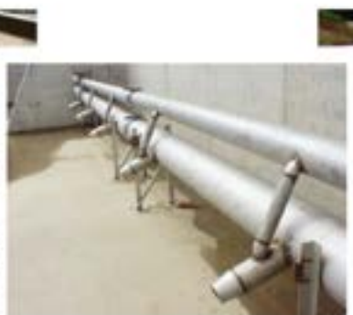
Independent Control of Oxygen Transfer and Mixing
