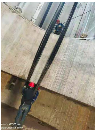
Install anchorage
