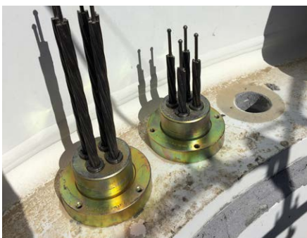
Install anchorage
