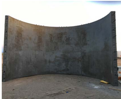
Cast tower section
