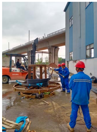
Manufacture cable coil
