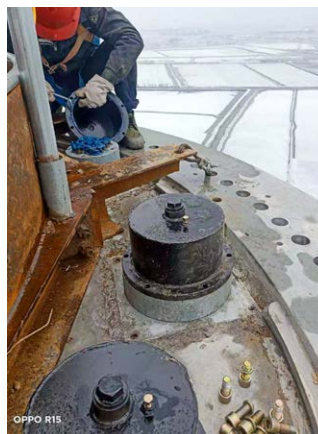
Prepare anticorrosion protection
