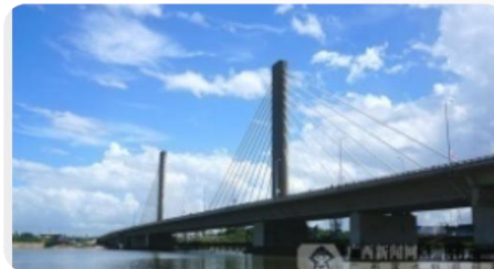
Kigamboni Bridge, Tanzania
