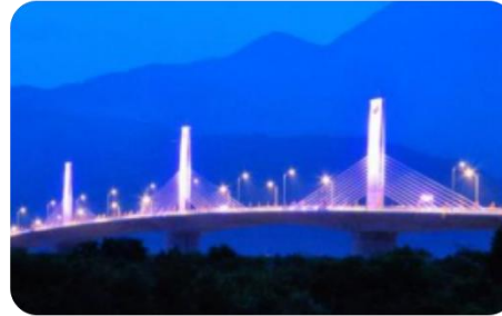
New Fengping Bridge, Taiwan Hualian
