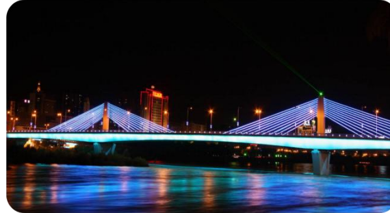
Lanzhou Xiaoxihu Bridge, Gansu
