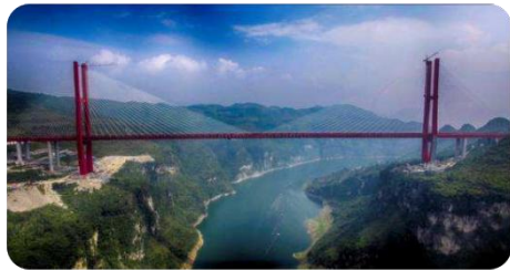
Yachi River Bridge, Guizhou
