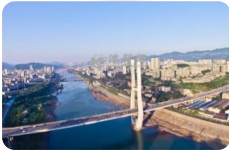
Jinshajiang bridge, Yibing Zhongba
