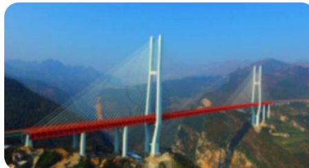
Bidu Expressway Beipanjiang Bridge
