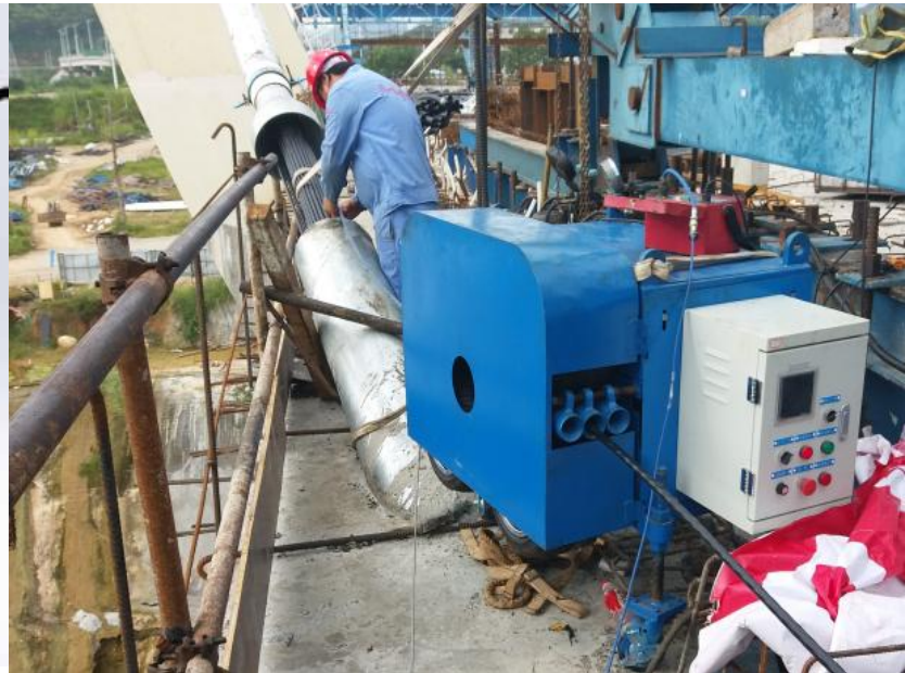
Patented Threading Machine for Extradosed Bridge
