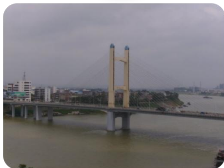
Liuzhou Huxi Bridge
