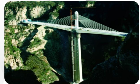
Xianshenhe Bridge, Jincheng, Shanxi
