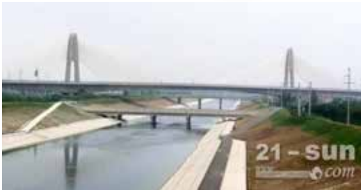
South-to-North Water Diversion Bridge
