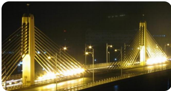
Zhangzhou War Preparation Bridge, Fujian
