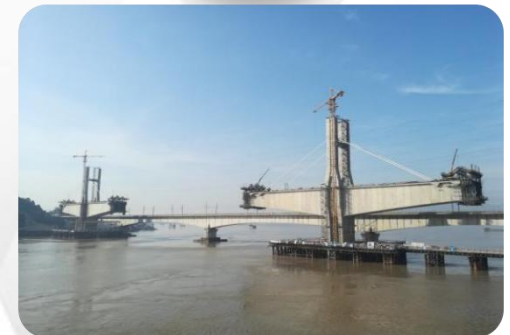
Wulongjiang Bridge, Fuzhou, Fujian
