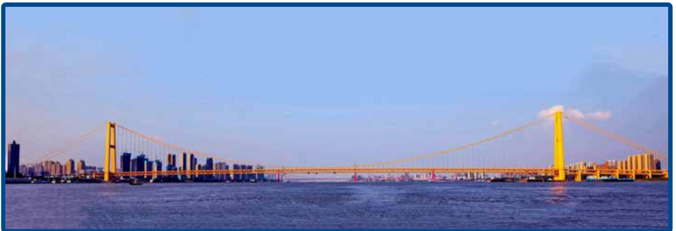
CHINA YANGSIGANG YANGTZE RIVER BRIDGE
