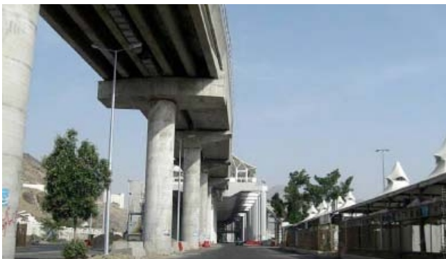
SAUDI ARABIA VIADUCT MINA-MUZDALIFA
