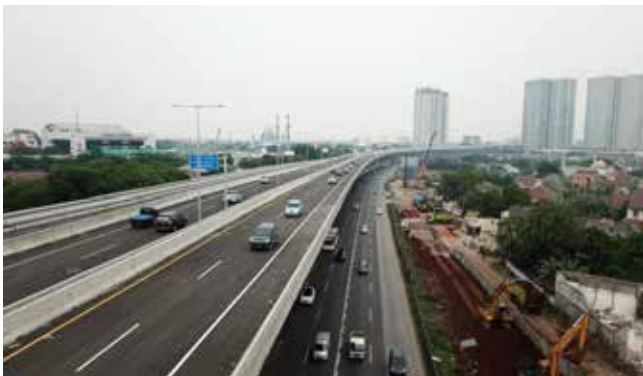
INDONESIA JAKARTA-CIKAMPEK II ELEVATED TOLL ROADS
