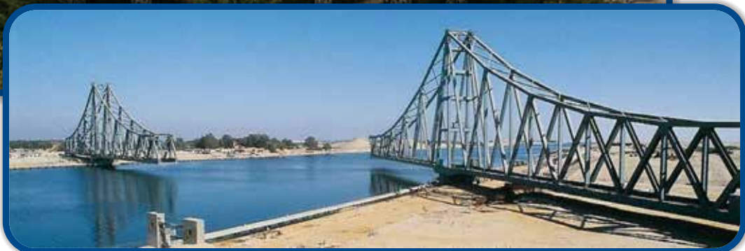
EGYPT EL FERDAN ► RAILWAY BRIDGE
