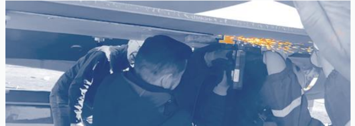
FIG. A: Quick and low-risk installation method tested in the ship repair yard at full scale.
