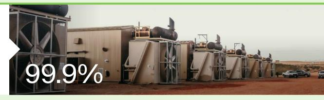
Crusoe's DFM™ technology converts the natural gas captured at oil wells and converts it into electricity by leveraging a stoichiometric combustion process, which allows reaching a 99.9% methane destruction efficiency.
