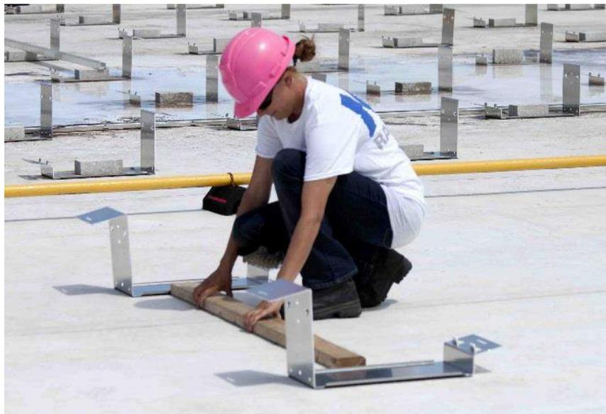
Figure 4 - Use of Spacer Sticks to Aid Placement
