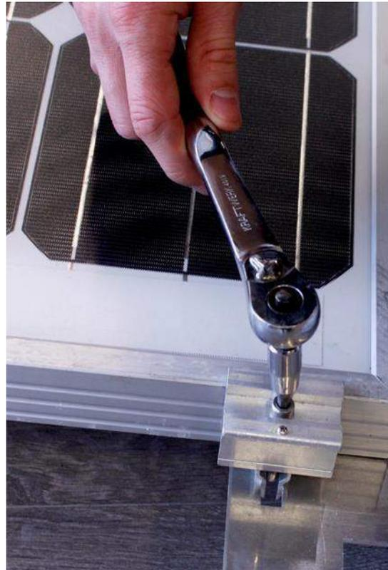
*Fig. 13 - Use Torque Wrench*
