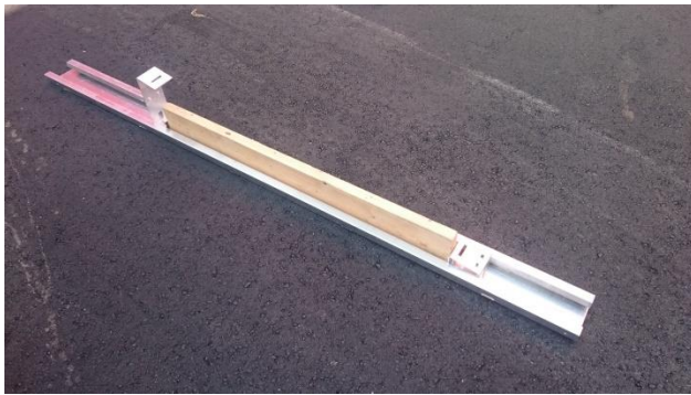
Fig. 12 – Use pre-cut wood spacers to evenly space supports
