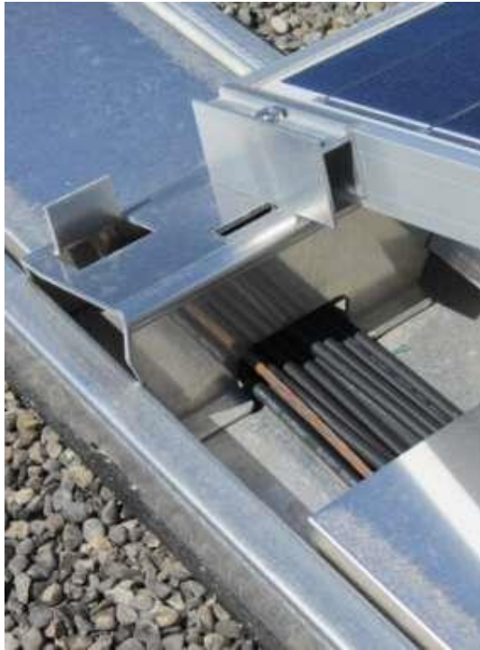
Fig. 25 – Rail cabling through supports
