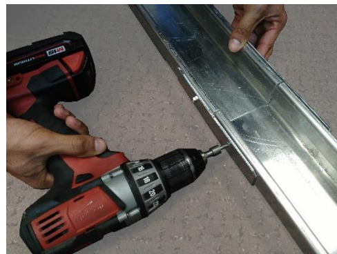
Fig. 5 – Connect two (2) Rails with Splice Plate
