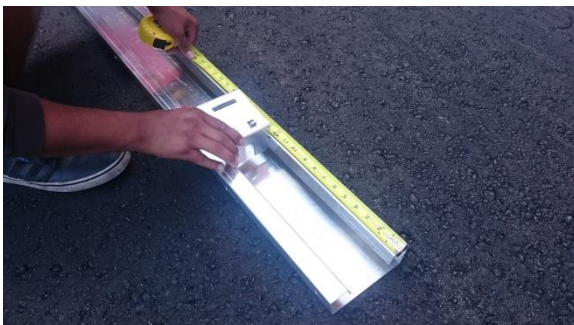
Fig.10 – Measure the first Bottom Support of the row
