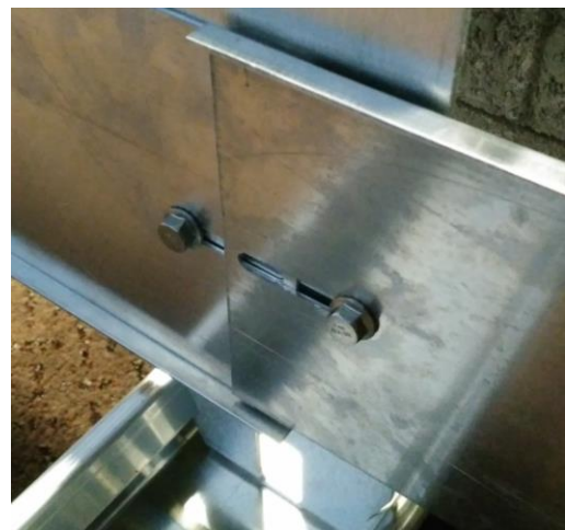
Fig. 27 – Torque shield to the Module Top Support
