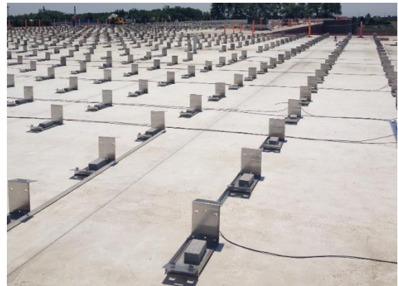
Fig. 2 - Supports Placed Prior to Ballasting
