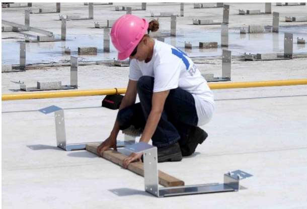
Fig. 1 – Use of Spacer Sticks to Aid Placement
