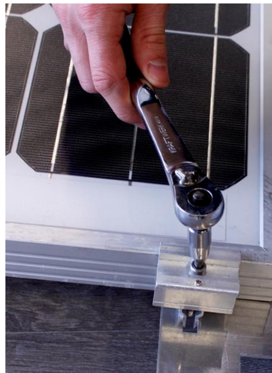
Fig. 12 - Use Torque Wrench
