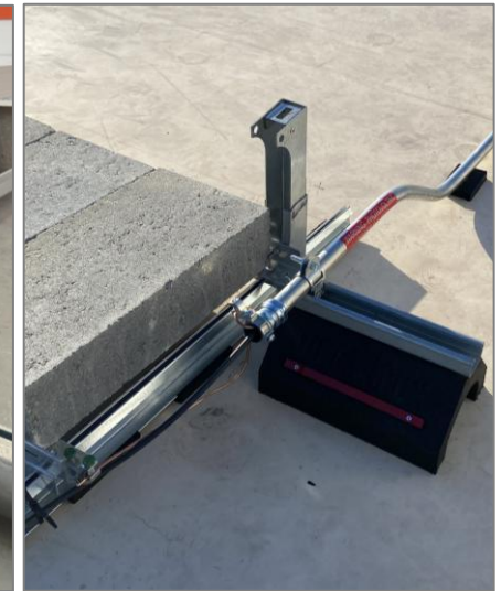
Example of Metal Conduit and Rooftop Support Block Along Array Edge
