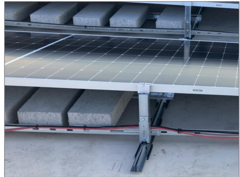
Example of Wire Management Along Ballast Trays with Wire Clips
