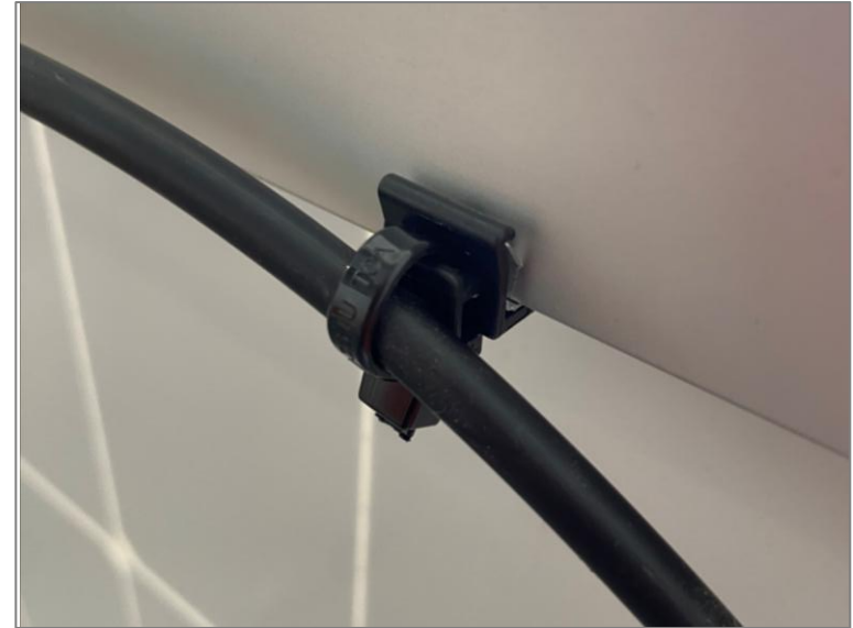
Example of Wire Clips Attached to Module Frame Flange
