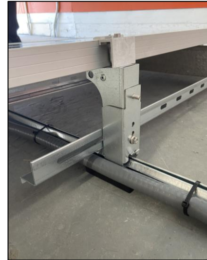
Example of Flexible Non-Metallic Conduit with Wire Clips
