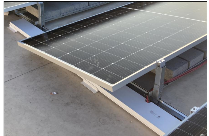
Example of RayTray Along Array Edge
