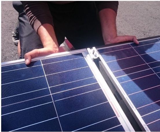
Fig. 23 – Two adjacent modules pulled together prior to securing clamp.
