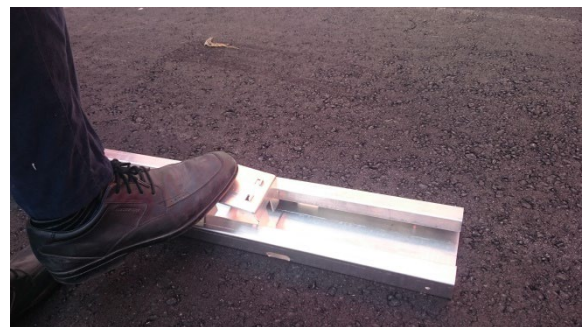
Fig. 11 – Click in the Module Bottom Support
