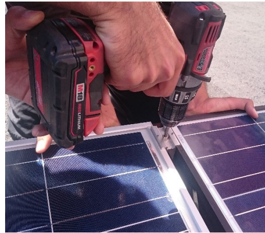
Fig. 24 – Two adjacent modules pulled together while securing clamp.
