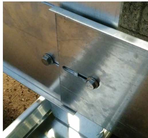
Fig. 27 – Torque shield to the Module Top Support
