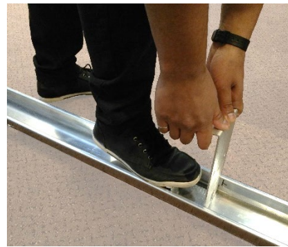
Fig. 13 – Click-in the Module Top Support
