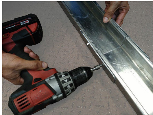
Fig. 5 – Connect two (2) Rails with Splice Plate
