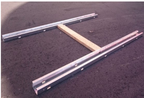
Fig. 2 – Use spacer sticks to aid placement
