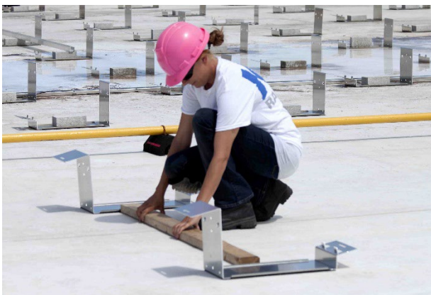
Fig. 1 – Use of Spacer Sticks to Aid Placement
