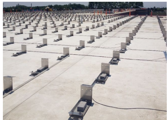
Fig. 2 - Supports Placed Prior to Ballasting
