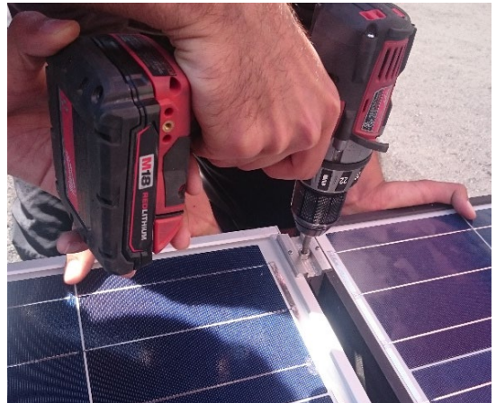
Figure 27 – Two adjacent modules pulled together while securing clamp
