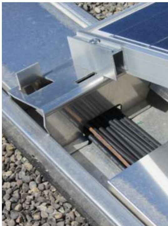
Figure 28 – Rail cabling through supports
