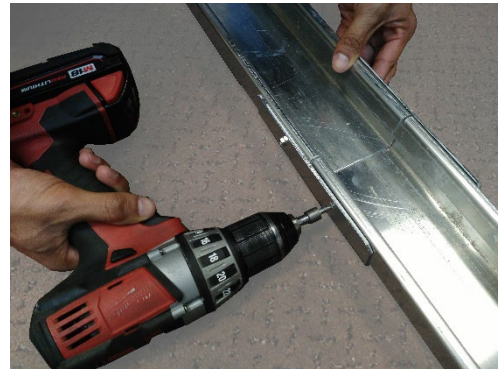
Figure 5 – Connect two (2) Rails with Splice Plate
