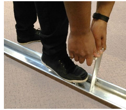
Figure 20 – Click-in the Module Top Support
