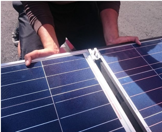
Figure 26 – Two adjacent modules pulled together prior to securing clamp
