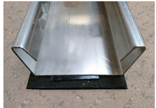
Figure 7 – Mat covers exposed Rail edge
