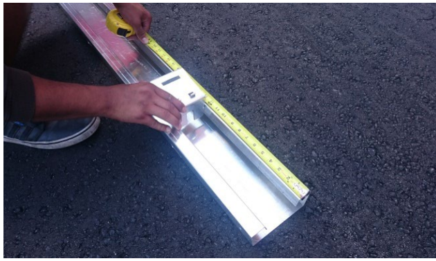
Figure 17 – Measure the first Bottom Support of the row
