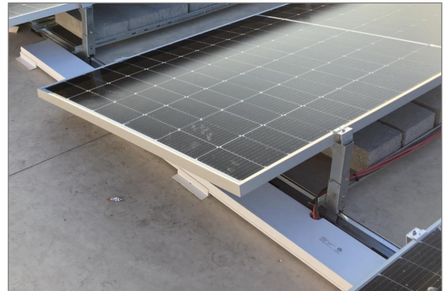
Example of RayTray Along Array Edge
