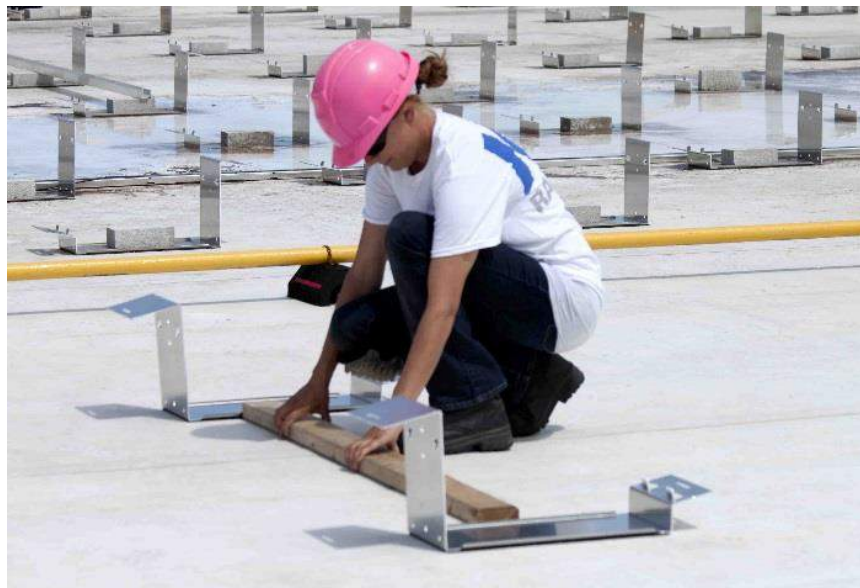
Figure 4 - Use of Spacer Sticks to Aid Placement
