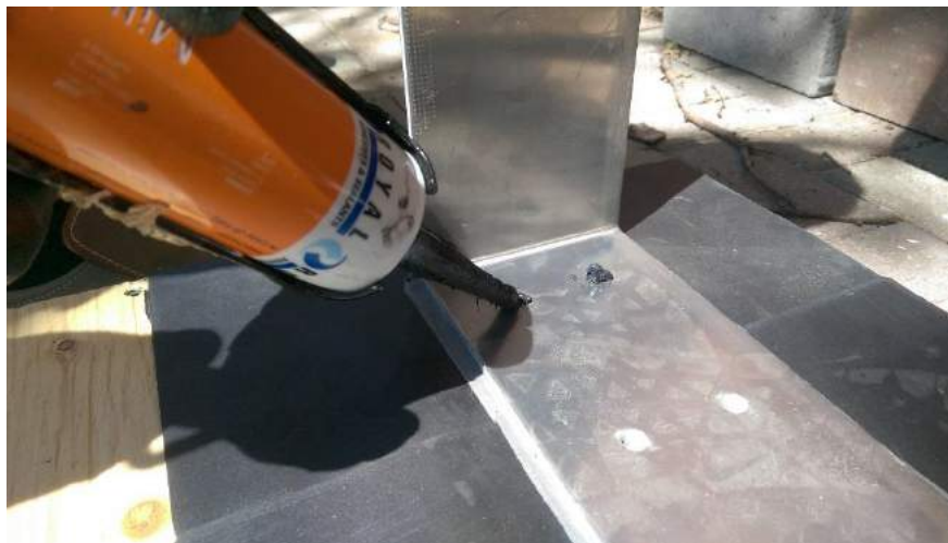
Figure 5 - Step 6: Apply LPS sealant on/in predrilled holes
