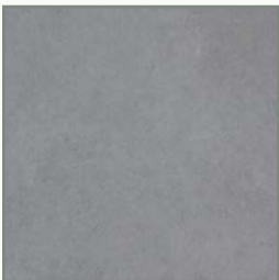
Driveway Smooth finished concrete
