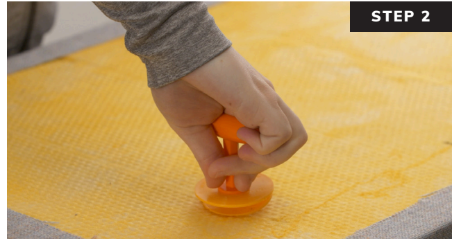
Screw Rotofast Snap-On Anchors into back of the panel using the Rotofast driver tool. Do not over-tighten.
