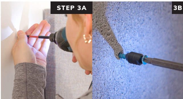
Screw black ratchets to wall at marked locations using the correct fastener for your substrate. Flat end of ratchet goes against the wall, curved end faces out.
