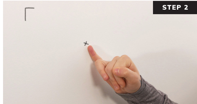
Mark the locations on the wall where the black ratchets will be installed in Step 3. For help with the number and placement of anchors, contact Rotofast.
