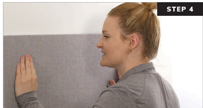
Push panel against wall to mark anchor locations.
