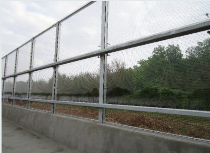
Example installation of a TL-4 System
