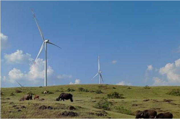
Kotada Pitha, Gujarat 16.2 MW wind | 9.8 MWp solar
