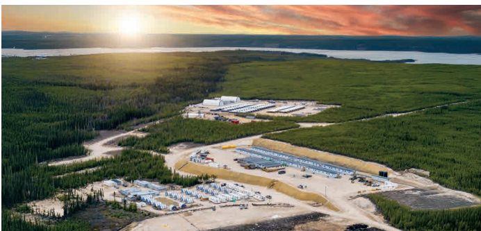
Rook I site in Summer 2024
