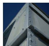
Sealing of cooling towers joints and seams
