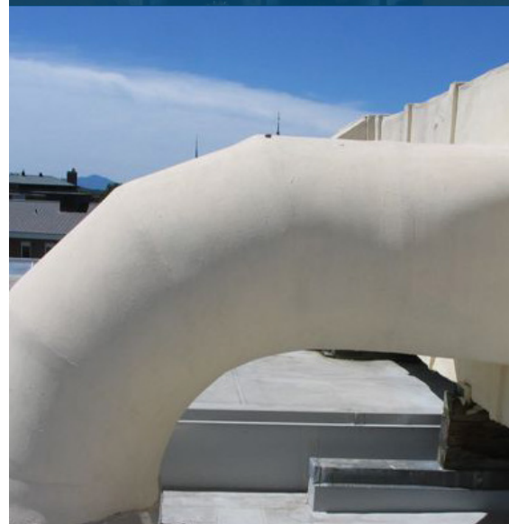
Protection against air and water ingress into ductwork
