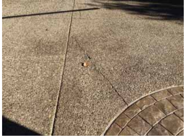
Concrete cracks
