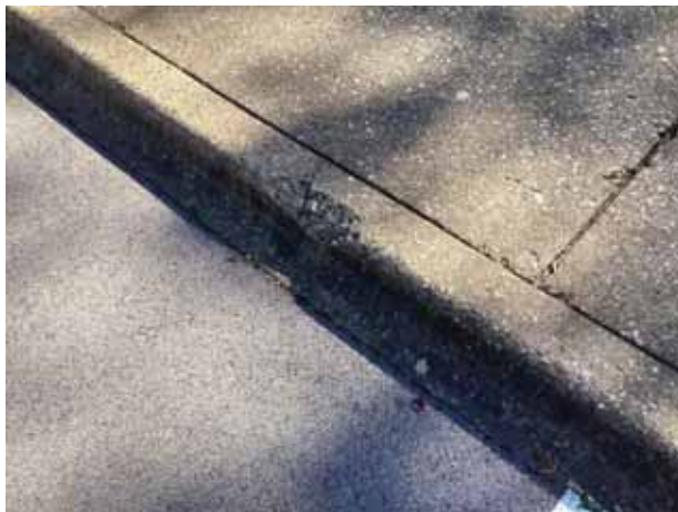
Concrete spalls
