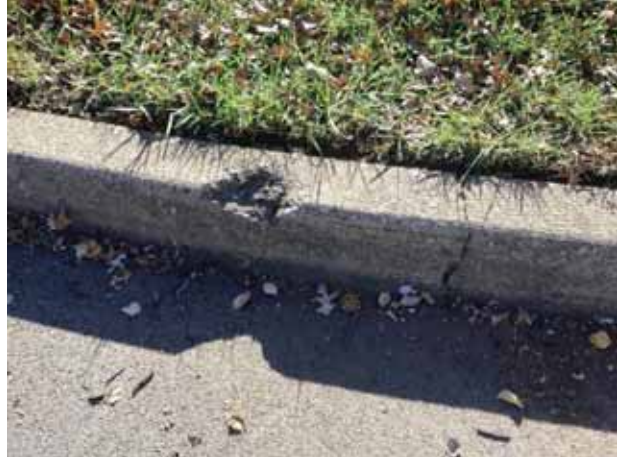
Concrete spalls
