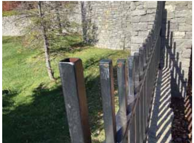
Missing fence cap and rust
