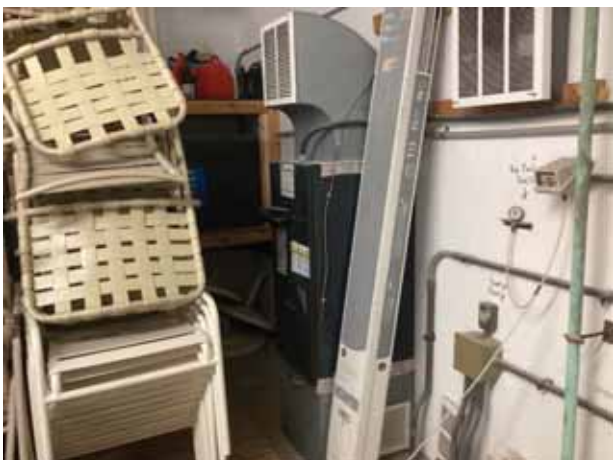
Split system air handling unit
