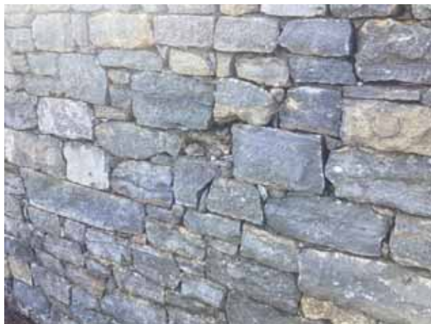
Masonry spalls
