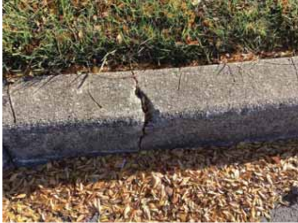
Concrete spalls
