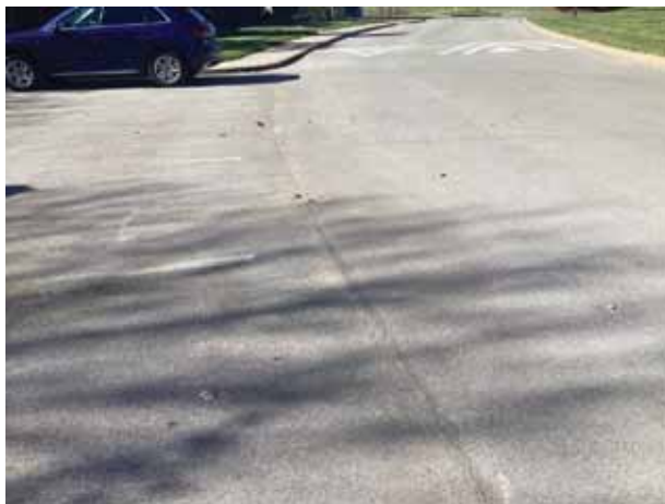
Pavement cracks
