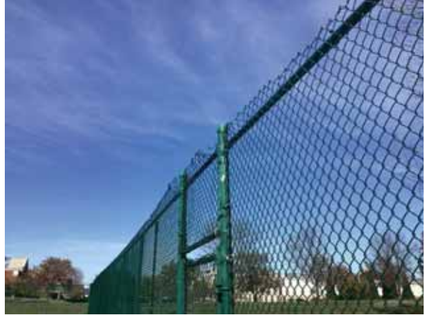
Fence warped webbing
