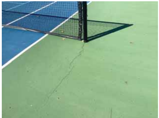
Surface cracks
