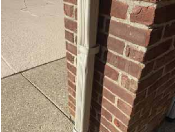
Downspout damage
