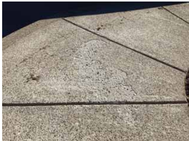
Sidewalk spalls
