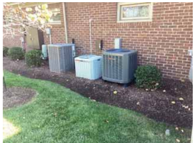
Split system condensing units
