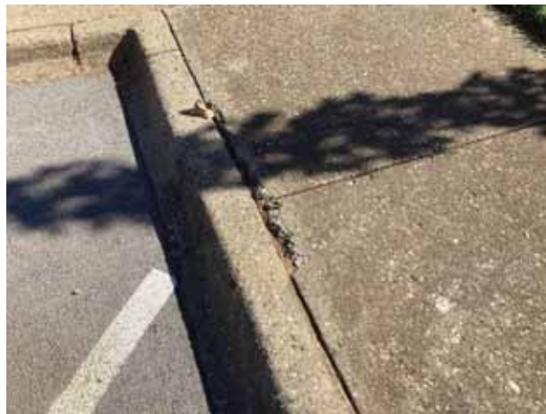
Sidewalk spalls
