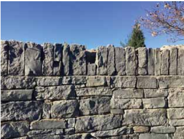
Masonry spall
