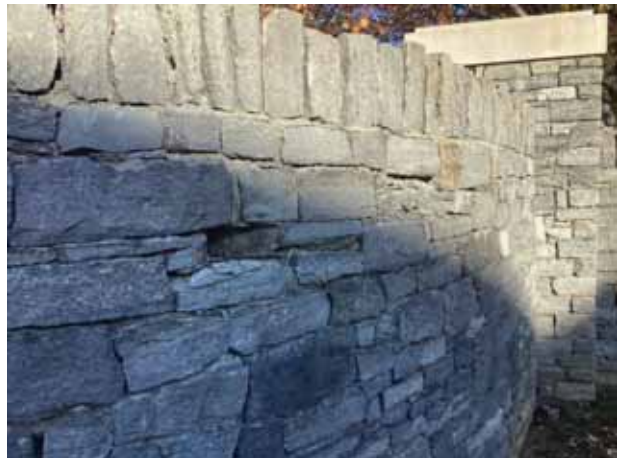
Masonry spalls
