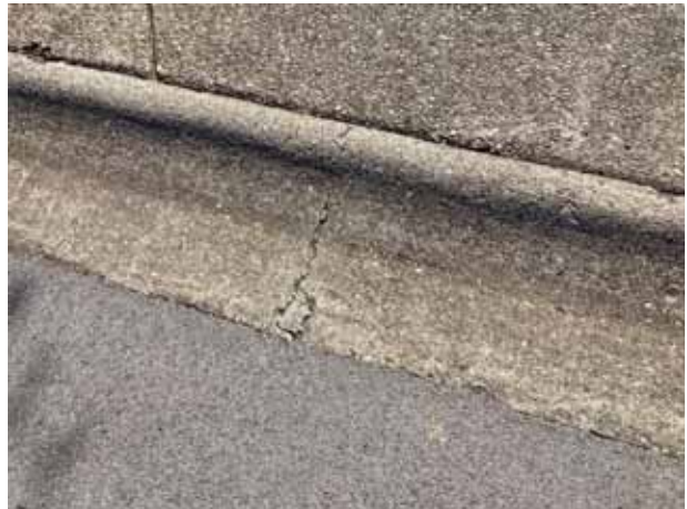
Concrete cracks
