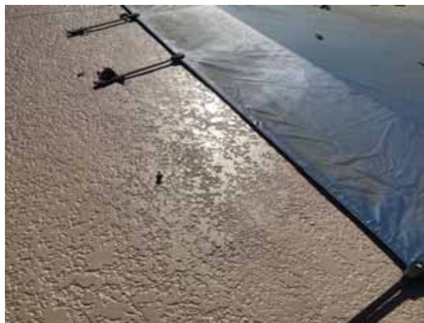
Missing pool cover connections
