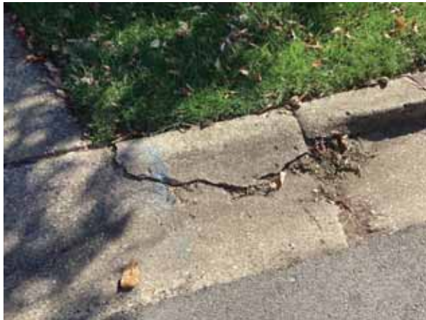
Concrete spalls
