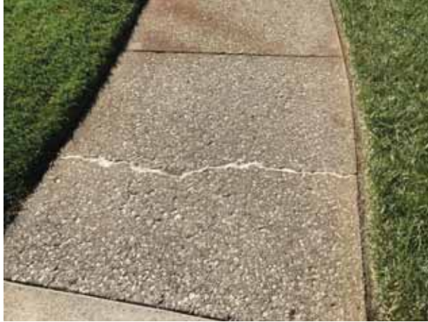
Previously repaired Sidewalk cracks
