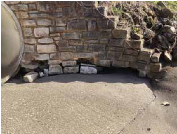
Masonry spalls
