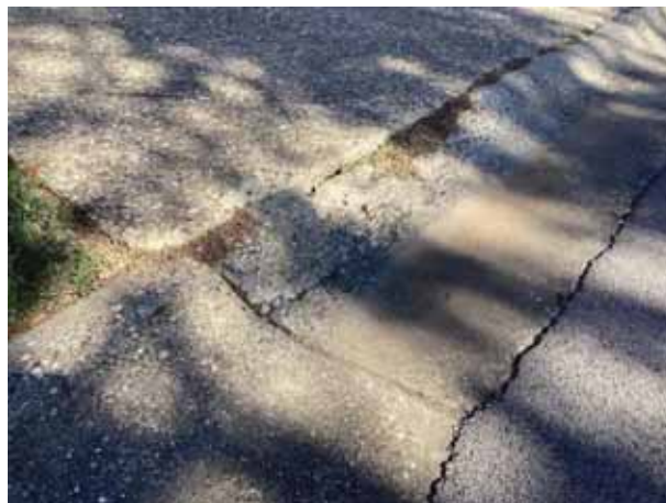
Concrete spalls (10108 Springhurst shown)
