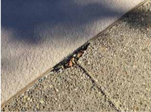
Concrete spalls
