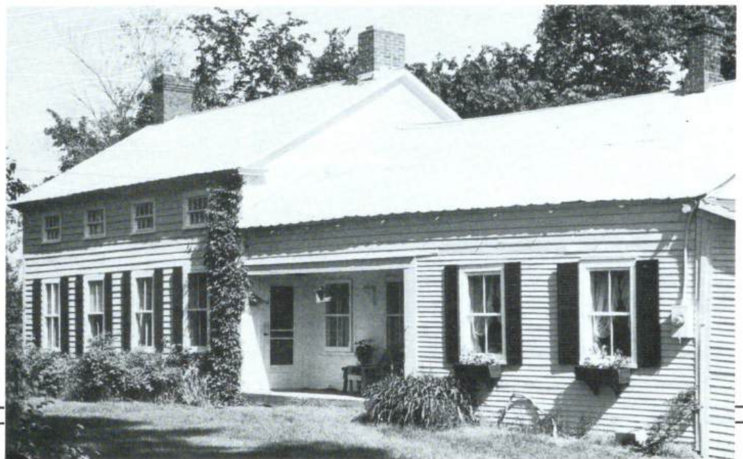
The Quaker Academy building as it appears today. It has been moved from the original location to its present site on Hallock Hill Road.
