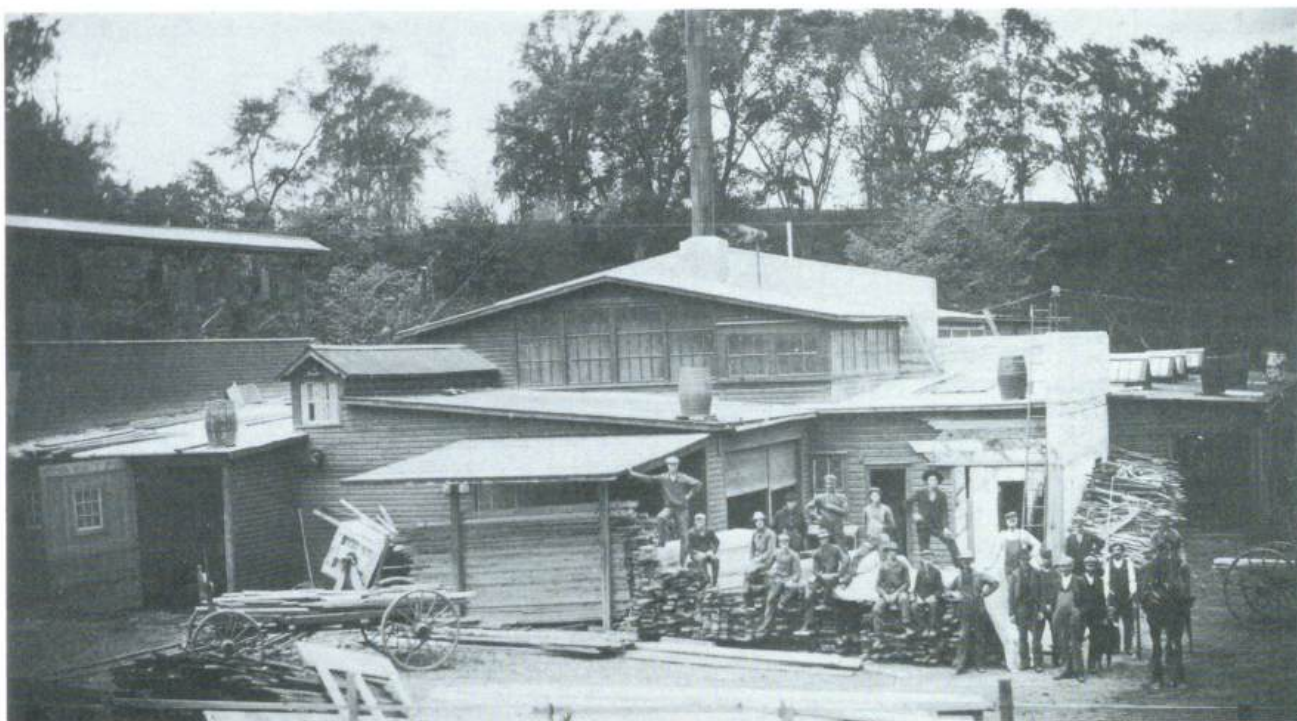
Mason's about 1908, when it celebrated its 25th anniversary. It had been enlarged and now showed some concrete walls for fire protection.
