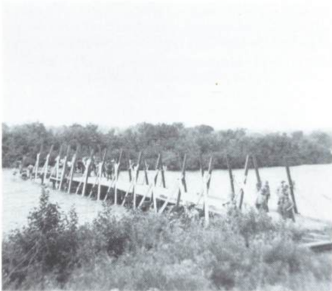
Engineers from either the regular army or the National Guard built a trestle bridge across the Saranac River near Morrisonville.
