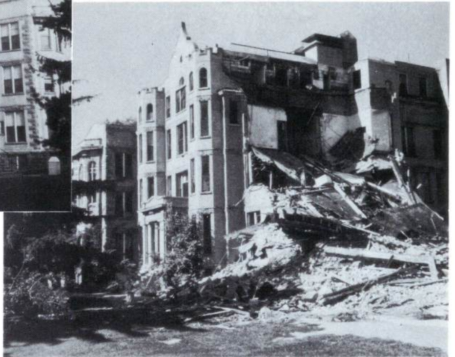
C.V. Hospital, partially demolished, 1978. Author's collection.
