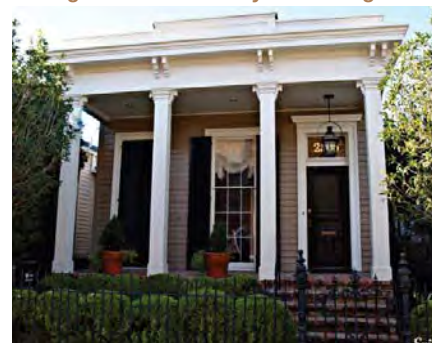
Cottage with vertically orientated windows
