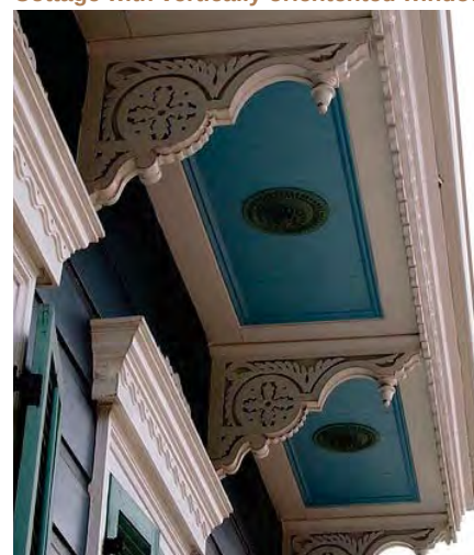
Overhang/Bracket detail at porch
