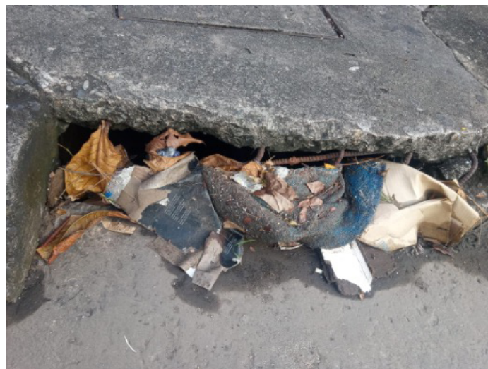
Figure 20: Example of storm drains clogged with debris and litter in the Mercado del Marisco area
