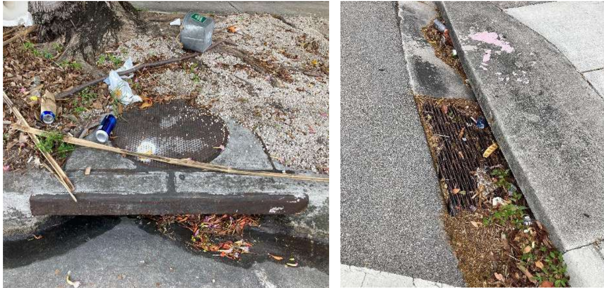
Figure 49: Example of storm drains in Miami without a grate or filter (left) and litter being stopped by an older version of a storm drain grate (right)
