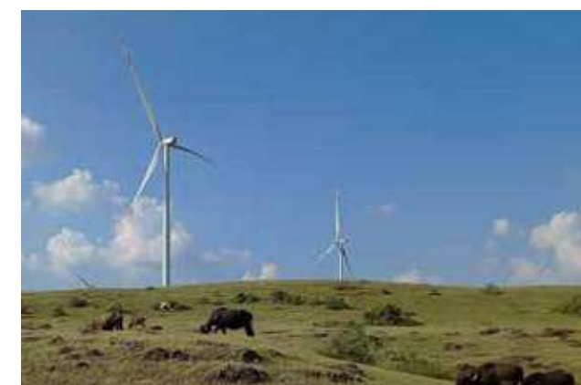
Kotada Pitha, Gujarat 16.2 MW wind | 9.8 MWp solar
