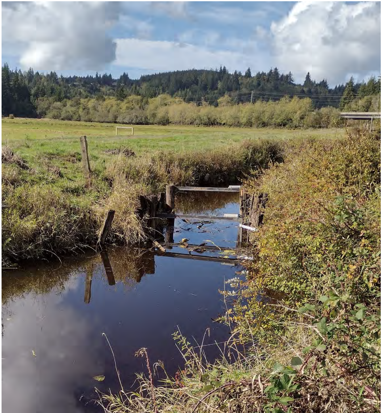
Figure 7. Double pass thru antennas installed on existing pilings of the westerly channel of Beaver Slough 100' above the tide gate.
