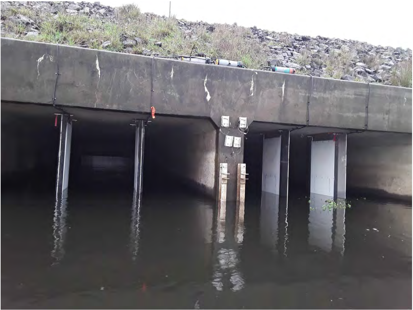
Figure 8. New blade style antennas installed on Gates 2B and 2C of Winter Lake Unit 2 in October of 2023.
