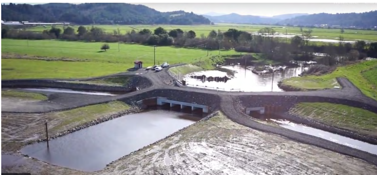
Figure 4. Aerial view of the landward side of the Winter Lake tide gate structures during construction phase.
