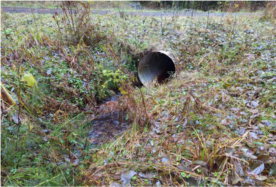
Photopoint 3: Culvert Site 2 Inlet 43.264404 -124.06935
