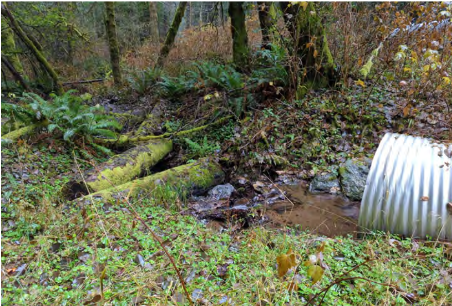
Photopoint 5: Culvert Site 2 Outlet From Side 43.26411 -124.06958
