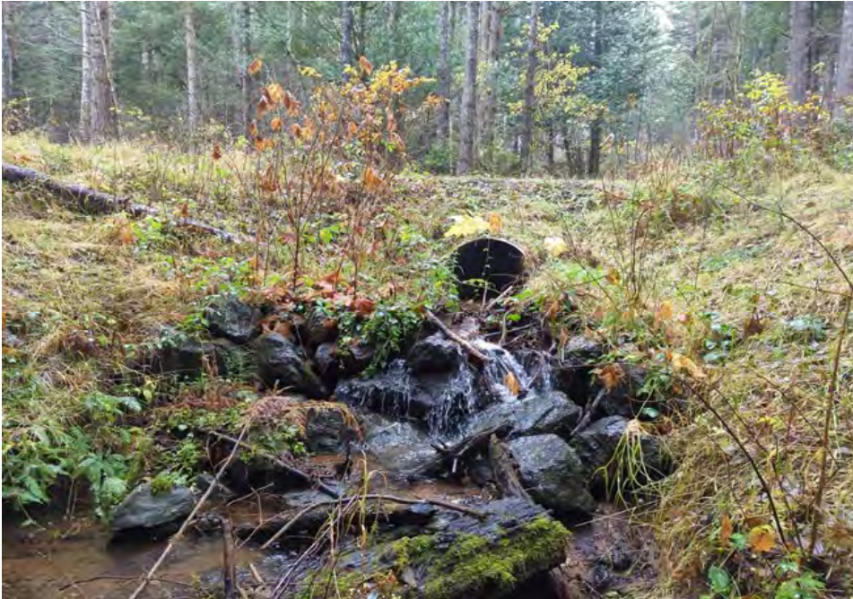
Photopoint 1: Culvert Site 1 Outlet 43.265240 -124.06817
