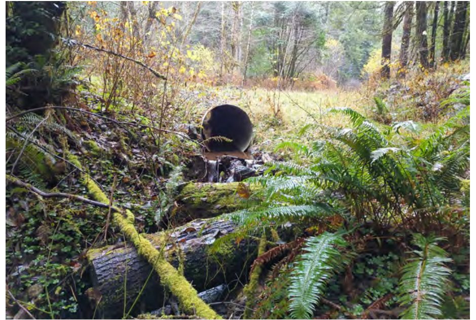
Photopoint 4: Culvert Site 2 Outlet 43.26406 -124.06951
