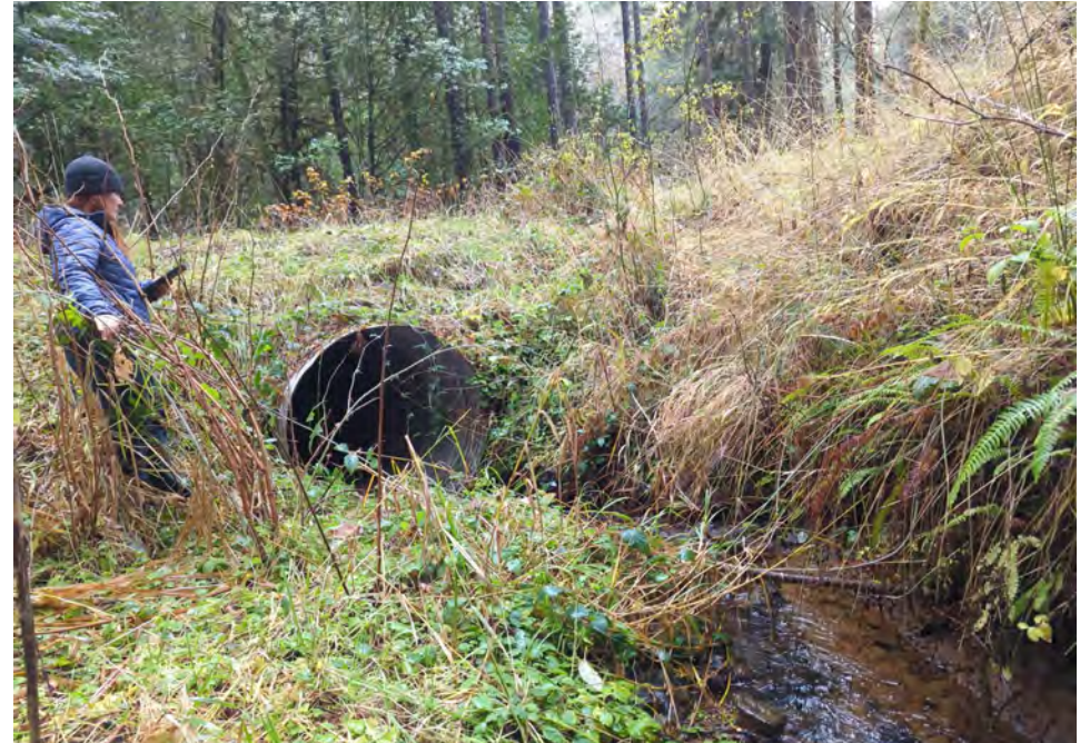
Photopoint 2: Culvert Site 1 Inlet 43.26556 -124.06833
