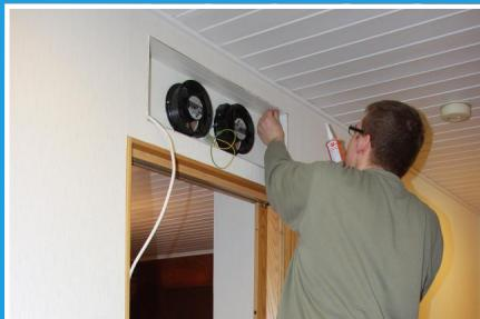
When the unit is installed into the opening, the edge of the wall structure and the passage channel is sealed. Direction of airflow is pointed towards the room that is to be heated / cooled.
