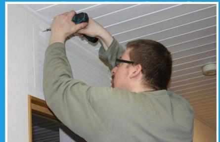
The grilles are fastened and the installation is complete. The grille is installed so that the airflow is directed up at the ceiling.
