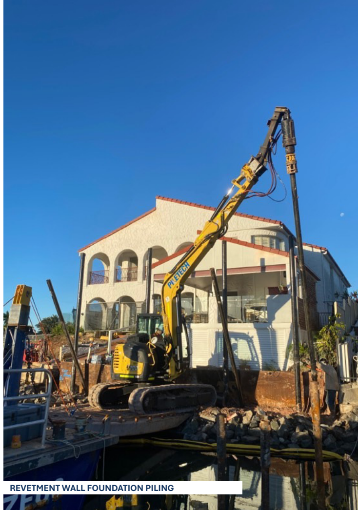
REVETMENT SLOPE STABILITY VERTICAL PILING
