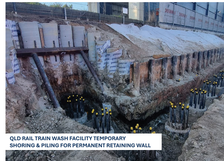
12MT DEEP X 750MM BORED PILES AT ROCKLEA TRAIN STATION
