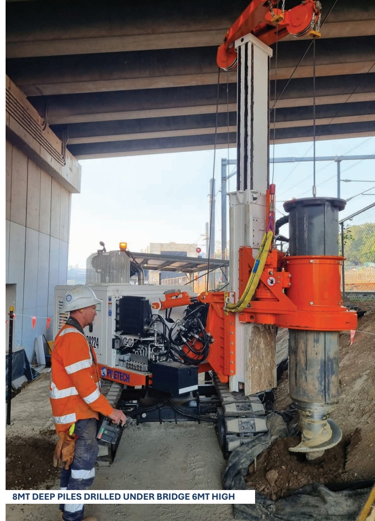
12MT DEEP X 750MM BORED PILES AT ROCKLEA TRAIN STATION
