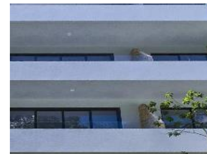
D White Paint Facade
